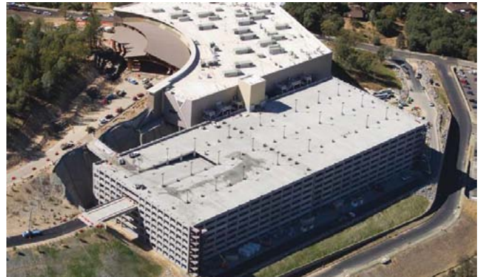
No. 18 Clark Pacific worked on the Red Hawk Casino parking structure in Shingle Springs.
