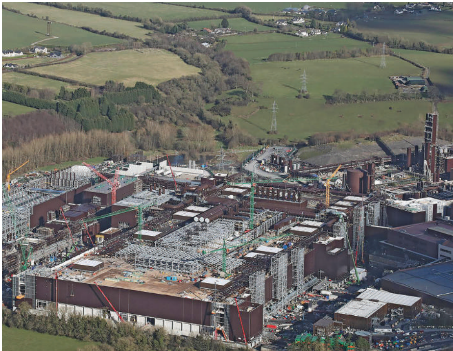
MAJOR EXPANSION Intel's under-construction Fab 34 would double its Irish manufacturing space.
