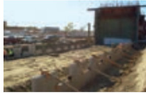
Cast-in-place abutment over I-405 features back-to-back Reinforced Earth walls.
