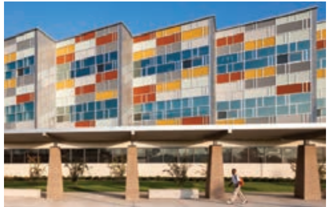
Helped by ARIDUS® Rapid-Drying Concrete, the energy-efficient Billy Earl Dade Middle School in Dallas was completed ahead of schedule.
