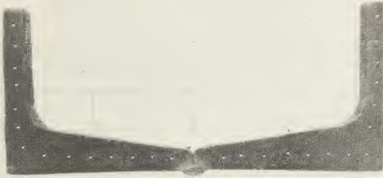
Figure A7.4.1-33 Transverse section 3Bm1 through the bottom of walkway box beam 9M (NBS 3). The south channel of the box beam is to the left and the north channel is to the right. The weld connecting the flanges of the two channels used to fabricate the box beam is in the center. Parts of the web regions of each channel had been removed before this photograph was taken. The indentations appearing on the surface of the section are the result of hardness measurements. Etchant: two percent nital. ~X1
